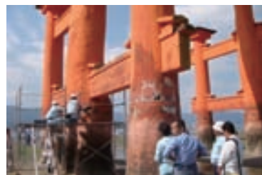
修復のための厳島神社大鳥居の調査 Examination of the torii of Itsukushima shrine for restoration
